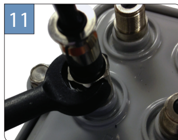
11 Tighten connector to recommended torque.
