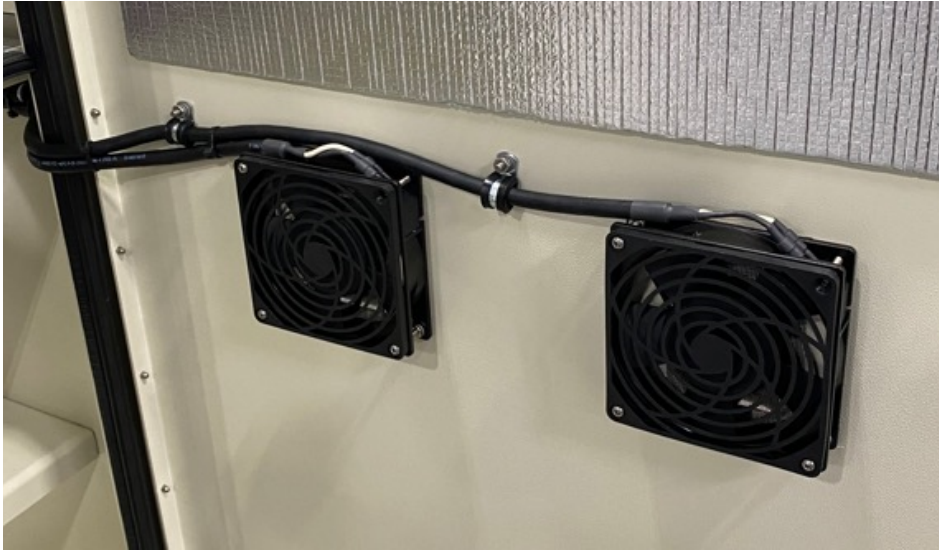
Figure L: Exhaust fans
