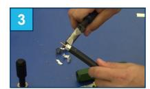
If using tri-shield cable, peel the exposed foil layer off, using pliers to assist if needed.
