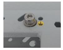
3.3. Insert the screw first through one washer, then through the M8 ring terminal of the earthing cable, and then through the second washer.
