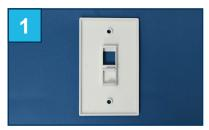
Align the wall plate in the correct position (the font on the back of plate indicates the correct upright orientation).
