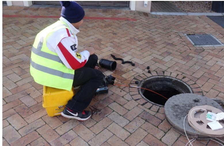
*Frogfoot installer deploying FTTH Miniflex through the drains*
