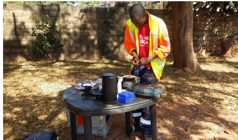
Liquid Telecom engineer preparing to install the PPC pre-populated aerial Dome
