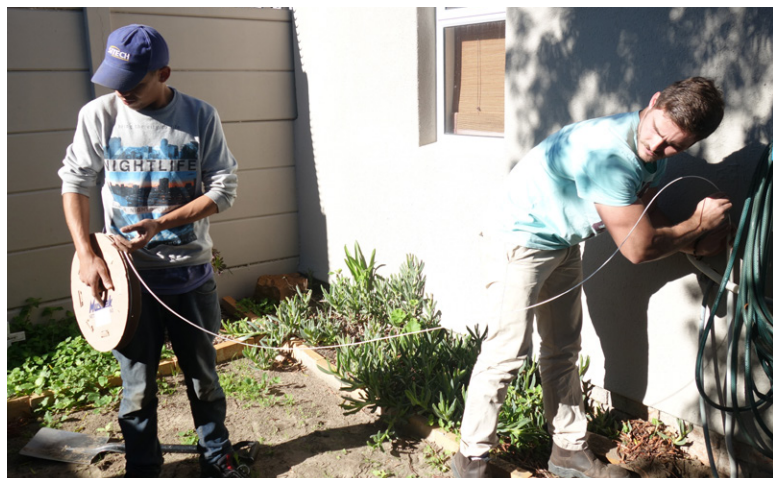
Hand-pushable Miniflex removes the need for expensive blowing equipment
