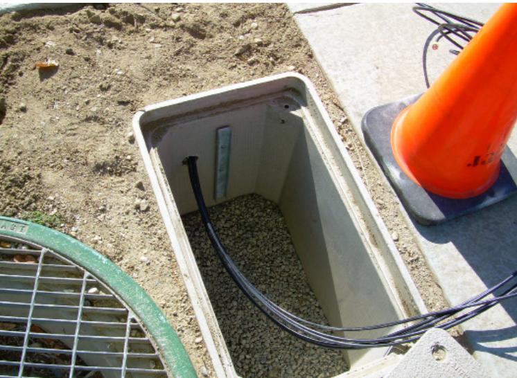
After evaluating the market for a solution, the city turned turned to PPC and adopted its patented Miniflex® pushable fiber cable and ruggedized TuffDuct® microduct, in combination with micro trenching, to bring down the cost and time of last-mile FTTP and FTTH deployments.
