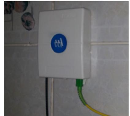
▲ Efficient and visually pleasing indoor termination to the customer premises wall box
