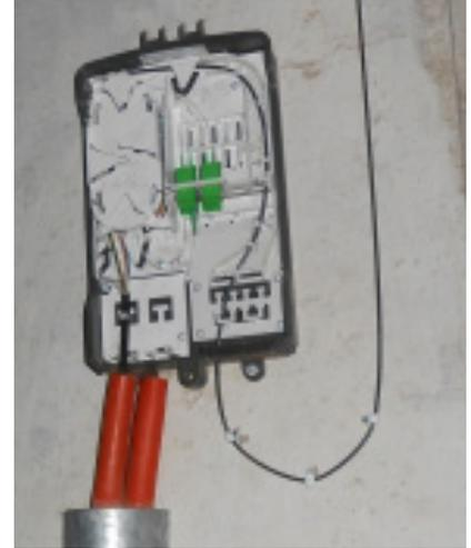
▲ Direct breakout from the ODB using Miniflex UV resistant fiber cable
