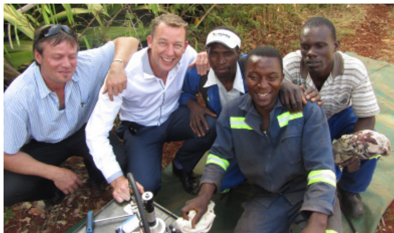
QuipHire Africa installation team installing at Liquid Telecom Zimbabwe customer premises
