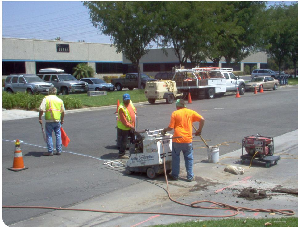
Utilizing pushable fiber, it is perfectly possible to push cable into a property in the space of a few minutes. Given that labor accounts for 80% of the cost of a typical FTTP deployment, this is a major advantage. And the technology can be deployed by non-fiber specialist engineers that have a limited knowledge of fiber optic installation.
